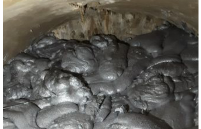
Geopolymer material during the installation process
